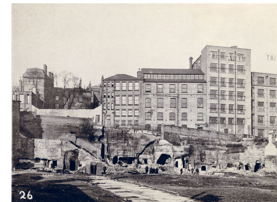
Red Lion Street demolitions, 1933 © Nottingham City Council, picturethepast.org.uk
